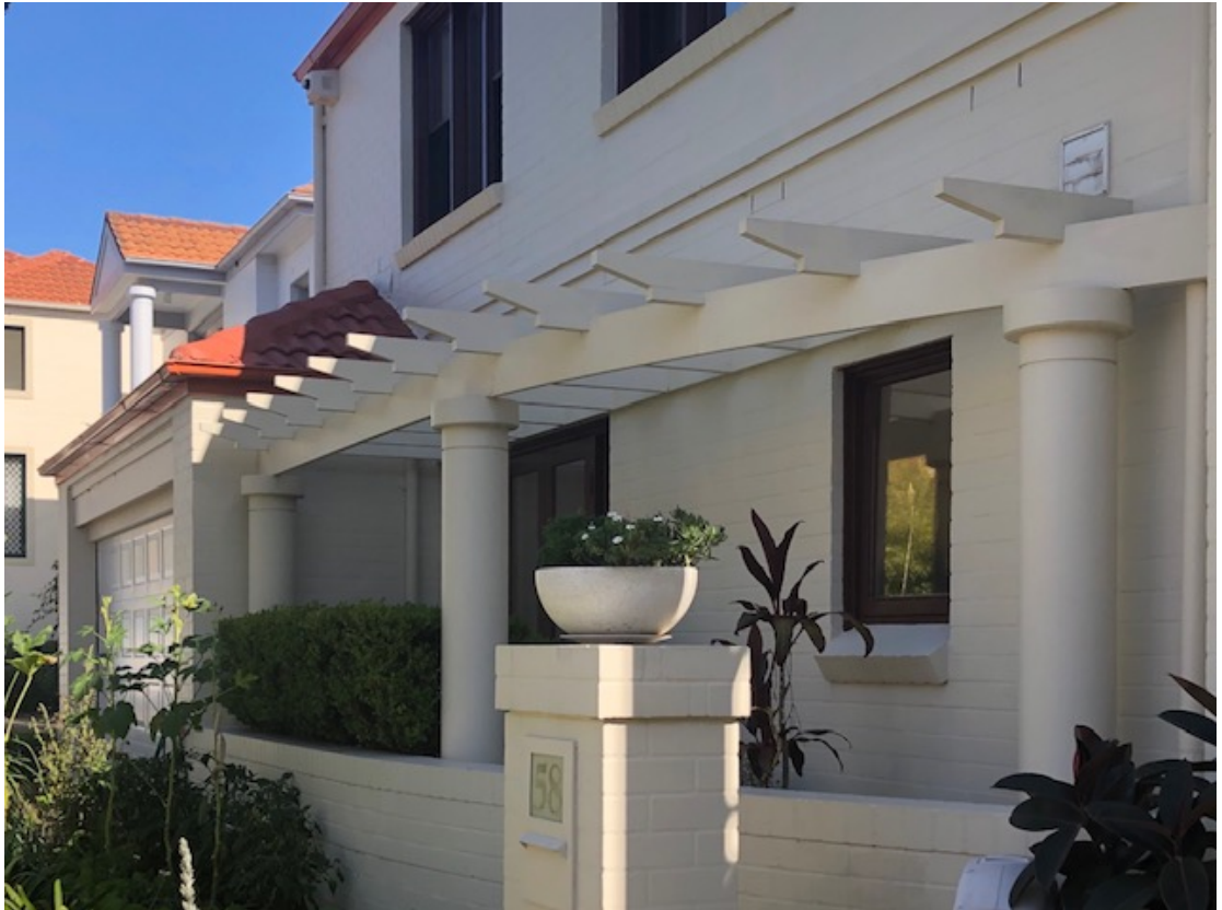
Pergola structure on house front aspect
